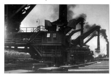
Hulett Ore Unloader bucket and men working inside bulk cargo hold
