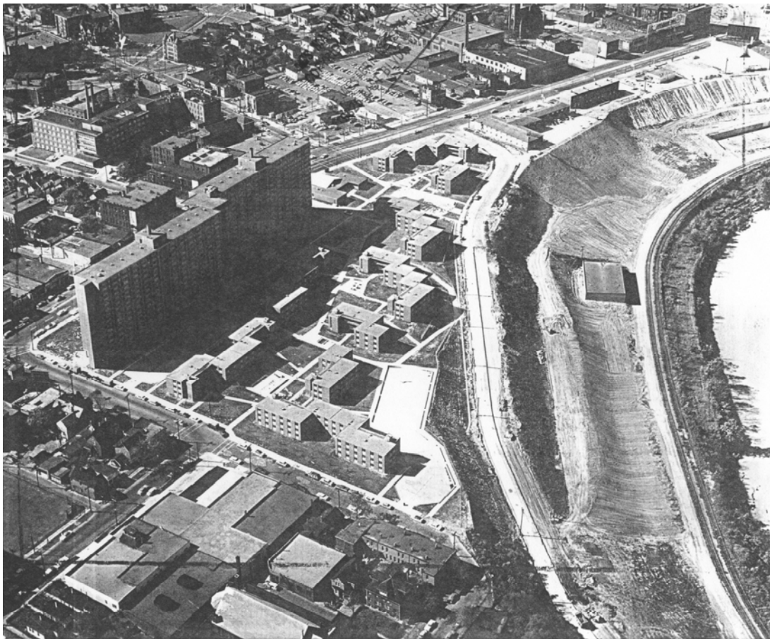
Image 5.3.4: Riverview Terrace 1963. Source: BBC&M Engineering, Inc
