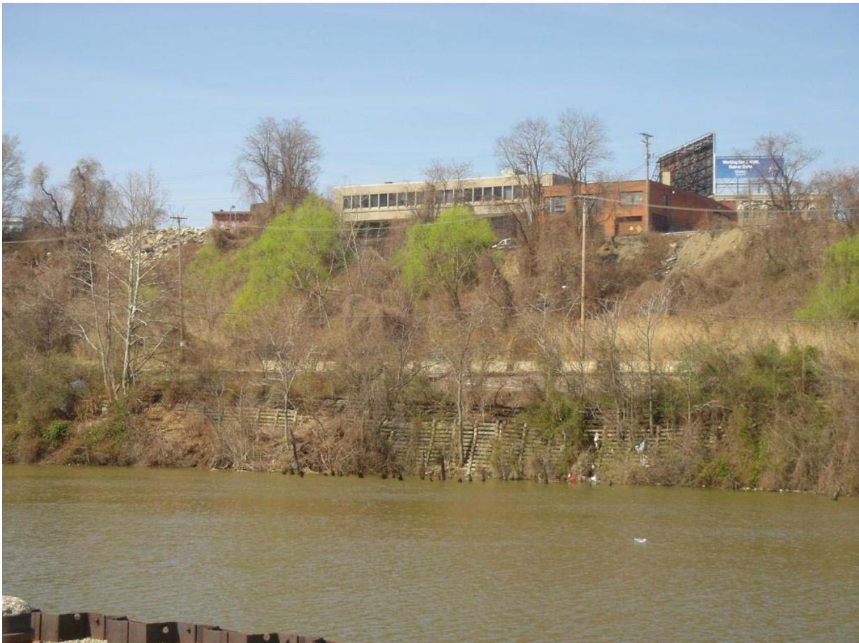
Image 6.1.1: Existing Cribwall. Source: USACE Field Inspection, 17 Apr 2008
