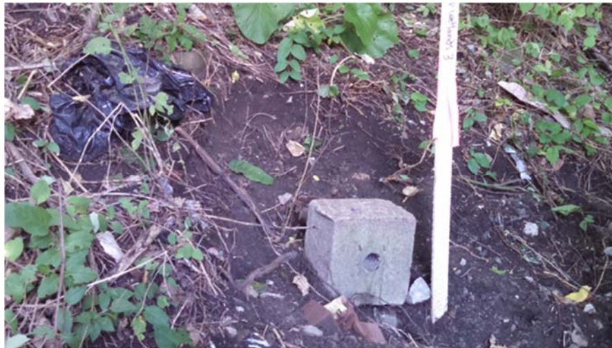
Figure 16: Horizontal 2" Diameter Drain Pipes Installed in 1966
