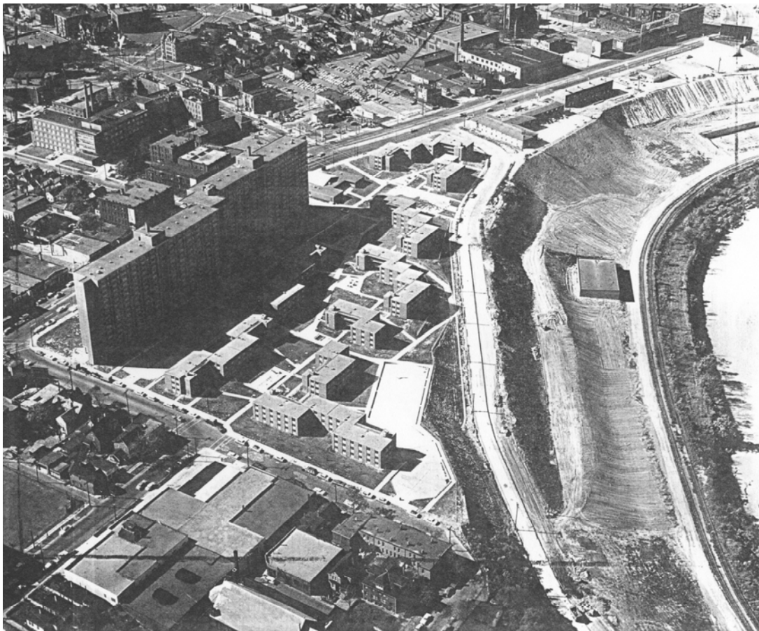
Image 5.3.4: Riverview Terrace 1963. Source: BBC&M Engineering, Inc
