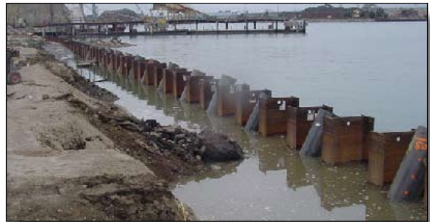
Port of Oakland, Phase 2
