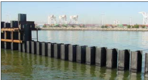
Port of Oakland, Phase 1
